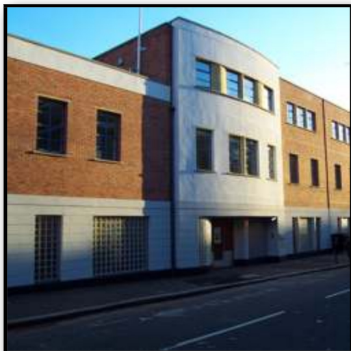
Front elevation from Hugh Street
