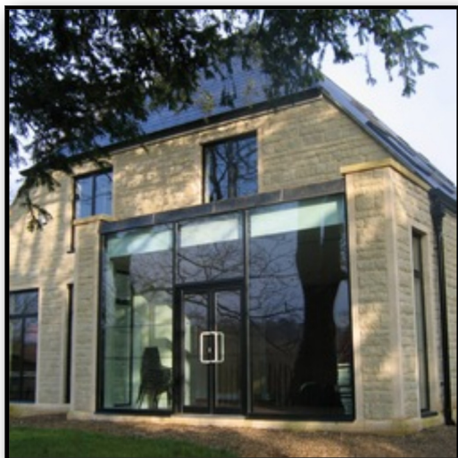
The church hall extension
