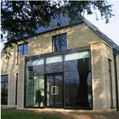
The church hall extension
