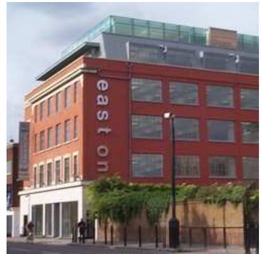
The front on Commercial Street
