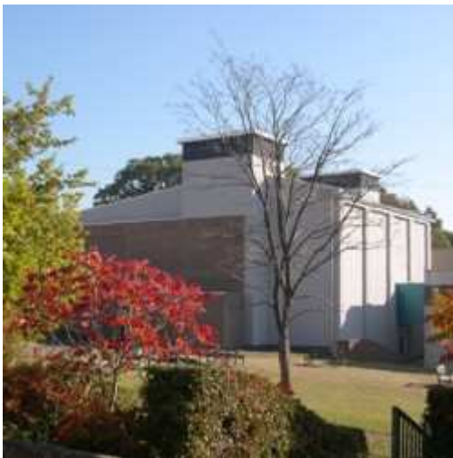
The ventilation towers
