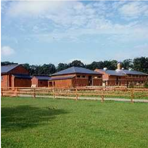
The stables of the Equine Centre
