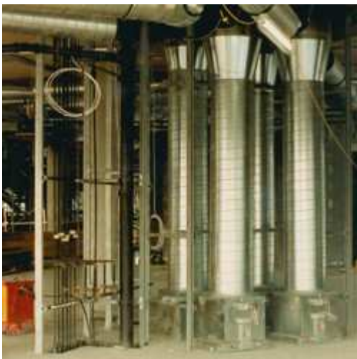
Ventilation ductwork under construction
