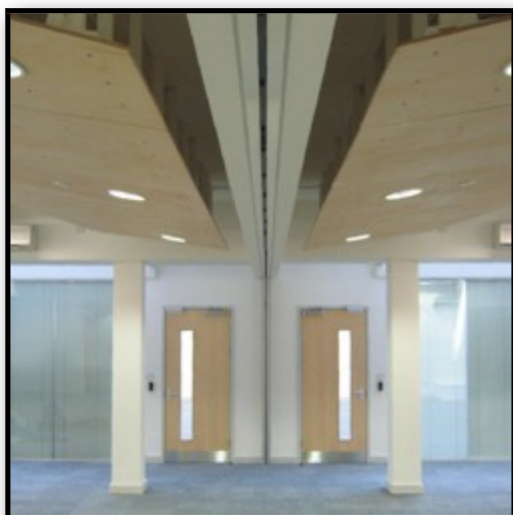
Acoustic Partition in Debating Chamber
