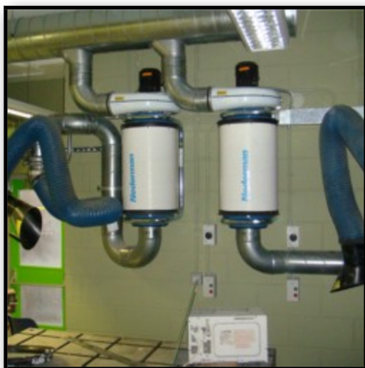
Local extract ventilation plant
