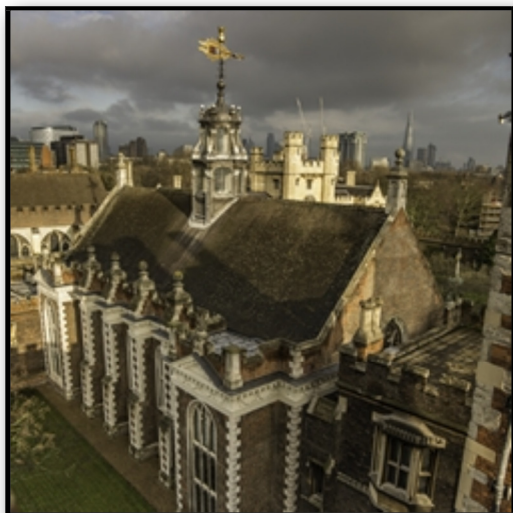
The roof of the Hall [Photograph Jonty M Sexton]
