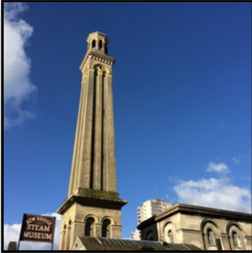
The iconic tower of the pumping station
