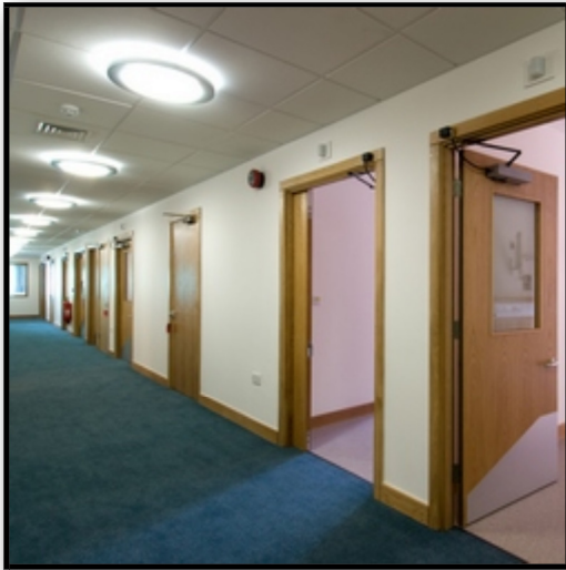
A corridor in the hospice
