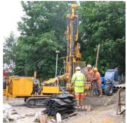
Drilling the GSHP boreholes
