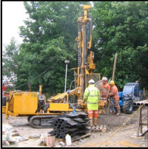
Drilling the GSHP boreholes
