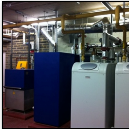
Inside the plantroom
