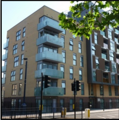
The exterior of Merle Court
