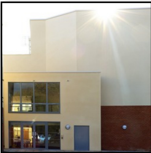
The new drama studios and theatre (Photograph:Ariane Teyssou/Tuke Manton Architects)
