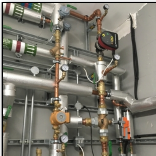
Heating pipework in the plantroom
