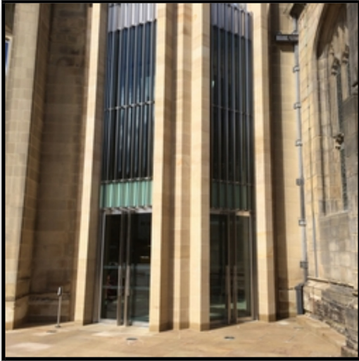
The welcoming new entrance
