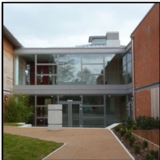
The exterior of the building
