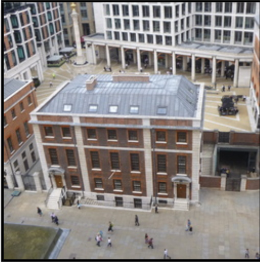
The exterior of the Chapter House, showing the restored roof
