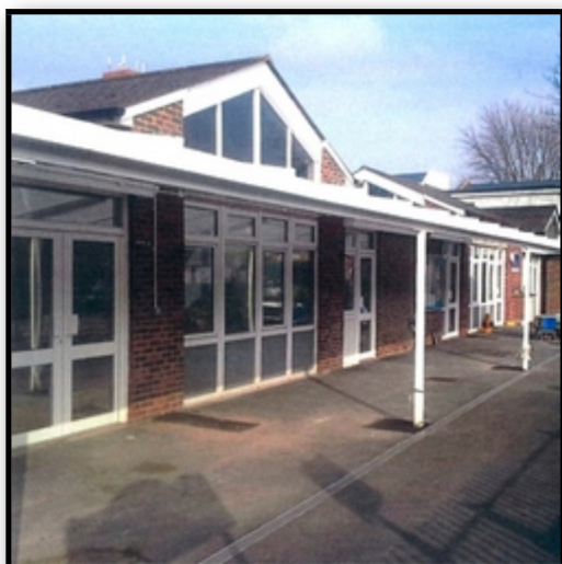
The newly completed school, with dormer window to the new mezzanine floor
