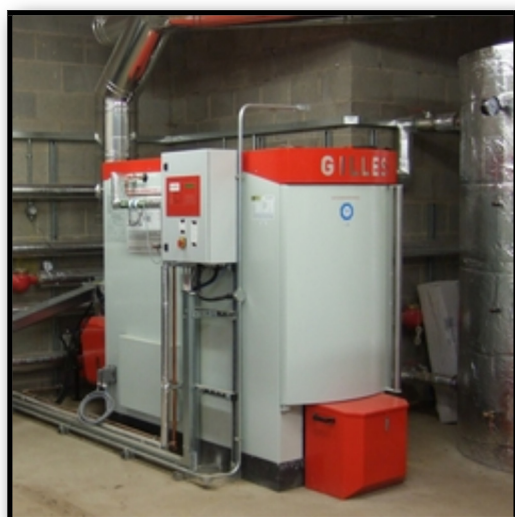
The biomass boiler
