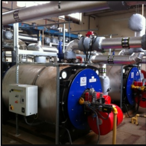
Boiler plant at the leisure centre
